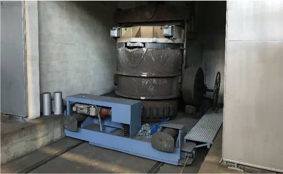
Fig. 8 Rail vehicles for the transport of melt
