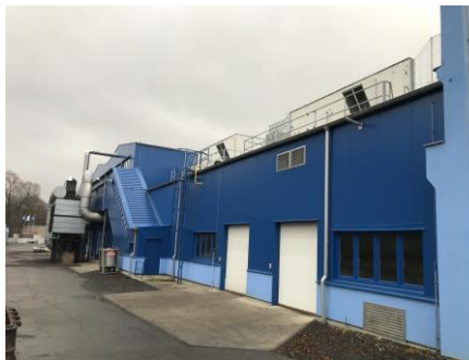
Metalurgie Rumburk, realization 2017 - 2020
