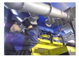
Inspection and replacement of damaged ducting, incl. complete deliveries of group I, II and III ducting.
